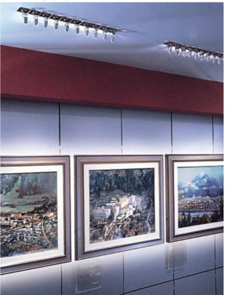
Conference room task lighting; five illuminators, each utilizing a 100W halogen lamp providing light to 288 lenses.
